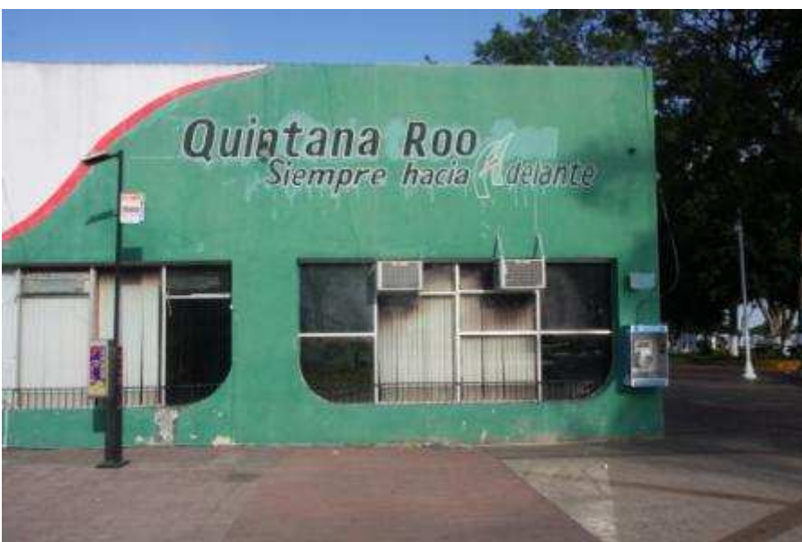
Administrative building Chetumal: "Always moving forward", but the state of the building...
