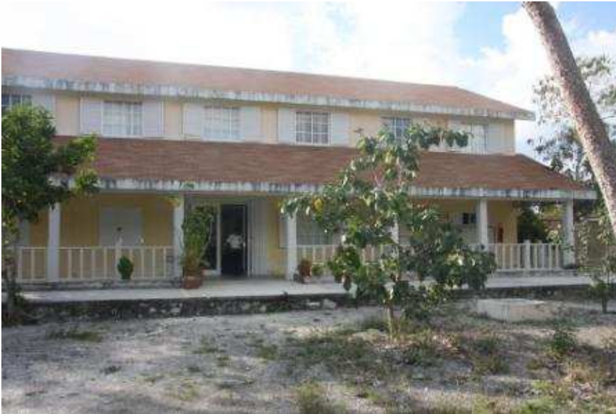
One of the teachers' buildings; the one where I share the office with Luis
