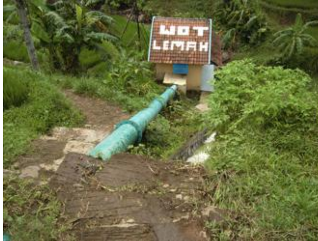
Image 5.1 Wot Lemah Micro-Hydro Plant.
