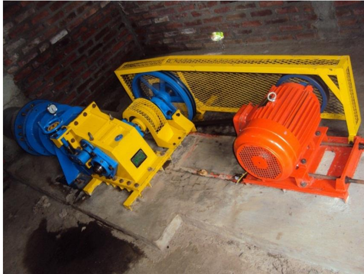
Image 10.1. Sendi MHP plant. We can observe a hole in the floor, near the generator (orange).
