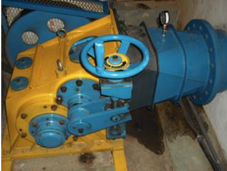
Image 4.1 Crossflow turbine T14 on Seloliman Micro-Hydro Plant
